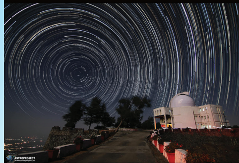
Mt Abu InfraRed Observatory (MIRO), Gurushikhar, Mt Abu, Rajasthan: Then (1990- no vegetation) and now: picture with star-trails (Courtesy, AstroProject), trees can be seen in front of the building.
